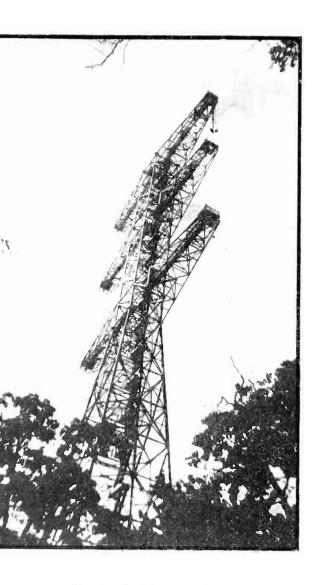
Four-hundred-foot steel tower Palisades supports turnstile antenna 900 feet above sea level. Radiating structure (see front cover) is supported between cross-arms at upper right
